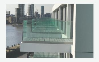
This means that when fitting the channel to an uneven surface, the angle of the channel can be countered by the adjustment of the glass.
